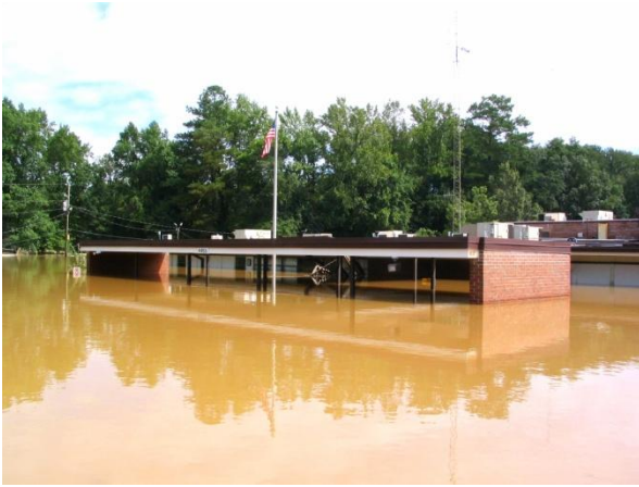
September 2009 Flooding at Clarkdale Elementary School
