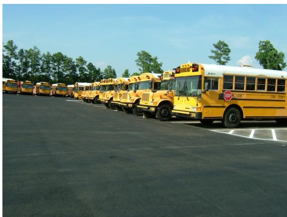
Bus Parking Lot Paving at Pitts Transportation
