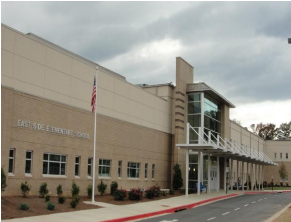
East Side Elementary Replacement School
