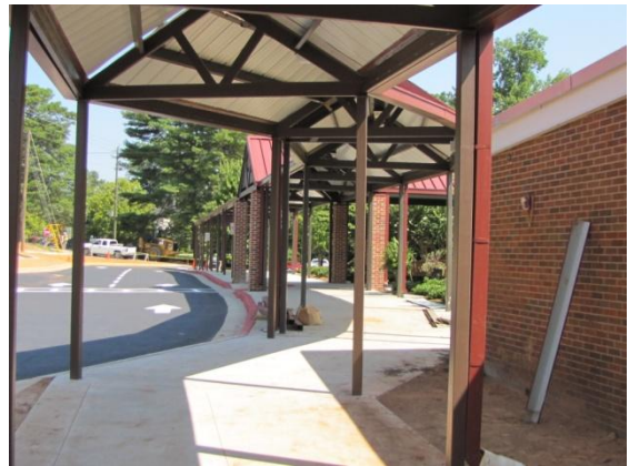
Driveway Modification at Teasley Elementary School
