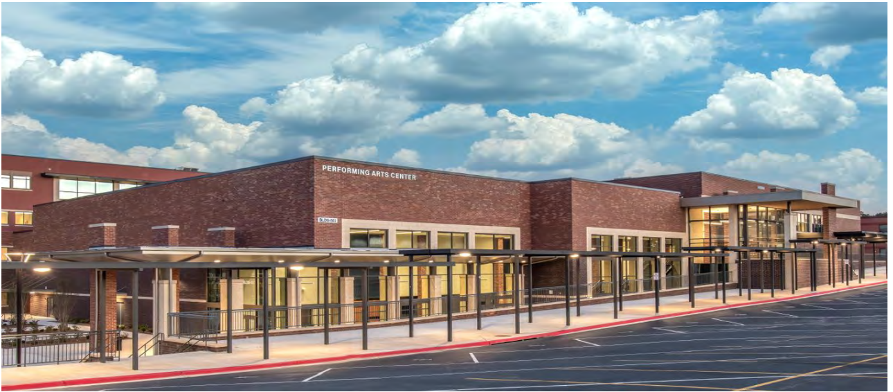
Osborne High School Performing Arts Center
