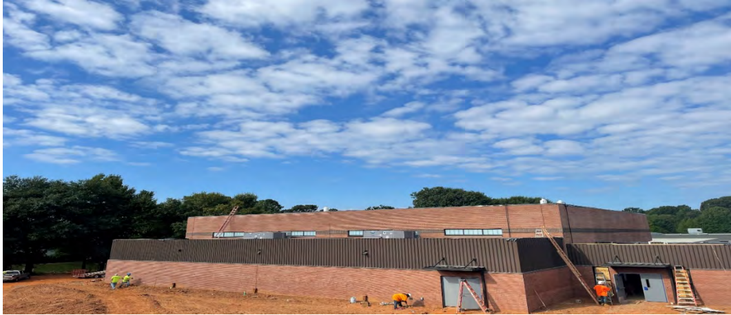
Sope Creek ES PE Building Renovation
