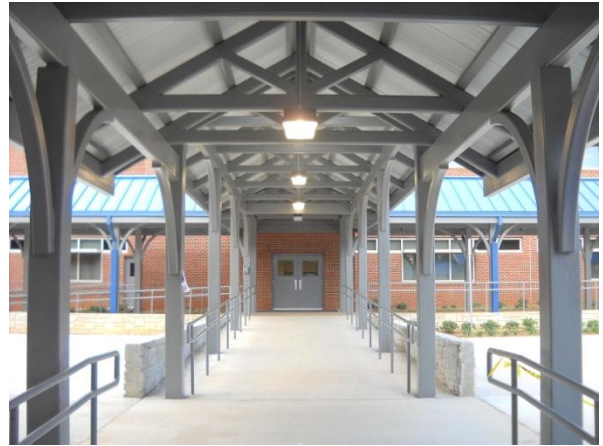
North Cobb High School Addition
