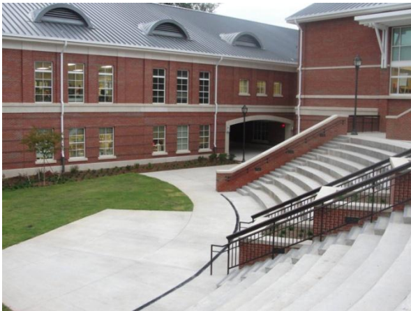
Mableton Elementary Replacement School
